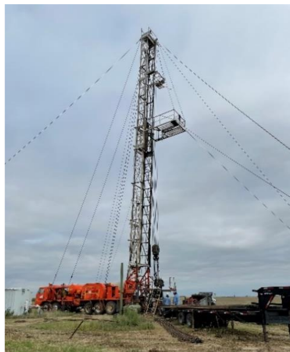
Figure 20. Well plugging in Deuel County, Nebraska.
